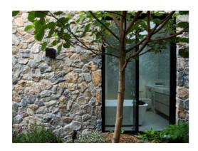
Stone cladding forms a layer around a structure to create a wall that appears like it has been built for century. In order to get the best outcomes, cladding should be installed by competent stone masons.
