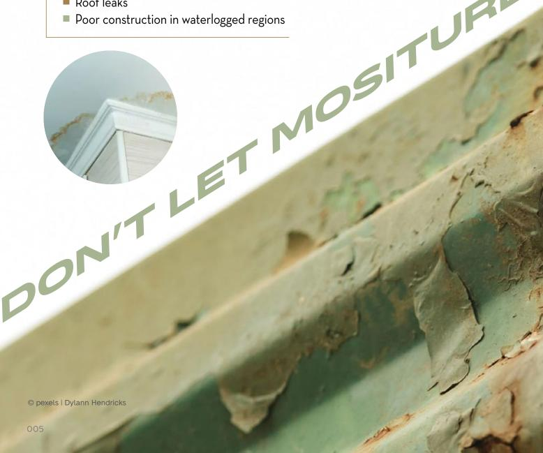
The effects of moisture in buildings, includes the possibility for damage to paint. This damage can cause paint to peel off uncontrollably. Furthermore, moisture can cause accumulation and build-up of moulds, fungi
